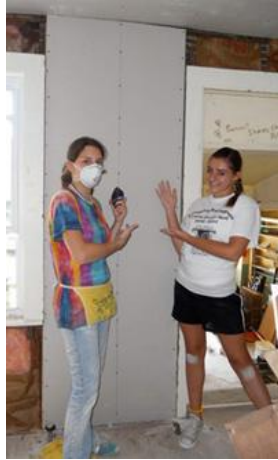
Putting up dry wall inside was part of the crew's job.
