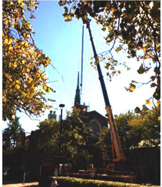
A crane is used to lower a liner into the First Church chimney on September 11. The liner was installed to make way for putting in a new boiler in the church lower level. The project is part of a busy autumn of work at First Church, made possible by the "Future's Broadening Way" capital campaign. See related article on Page 2.
